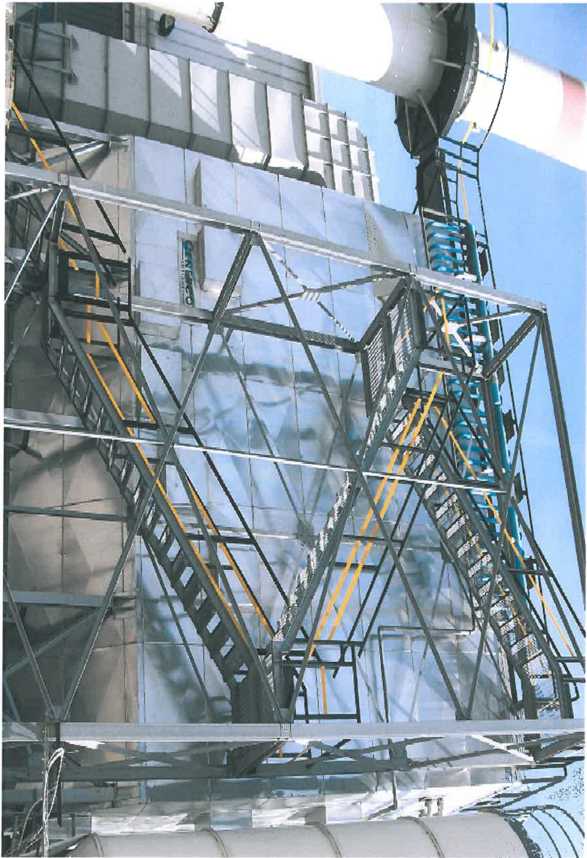
DRY CHANNEL ASPIRATION
